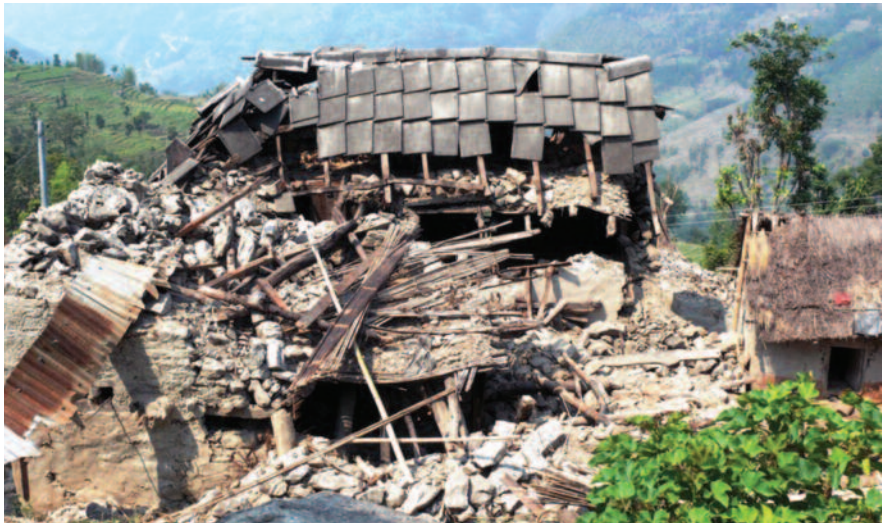
Traditional house built of stones, mudbricks, wood and slate stones for roof cover, Nepal. Photo by Per Andersson, 2015
