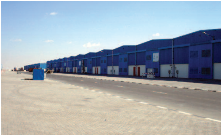
The photo shows the UNHRD Warehouses in Dubai. Photo by Martin Dalton, 2015.
