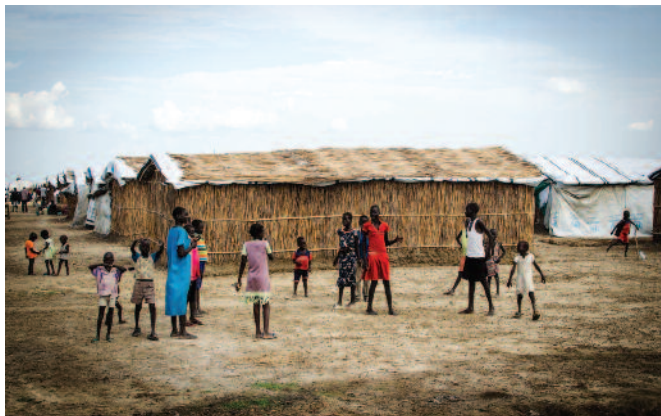
The photo shows Children playing outside a newly constructed Robust Emergency Shelter in the extension area, Benitu Camp, South Sudan. Photo by Colm Moloney, June 2015.
